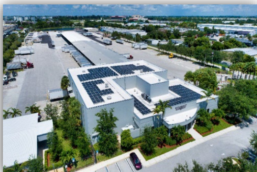
Ft. Lauderdale, FL System Size: 122 kWdc Commissioned in 2021 Net-Metered
