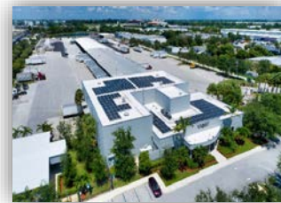
■ Ft. Lauderdale, FL System Size: 122 kWdc Commissioned in 2021
