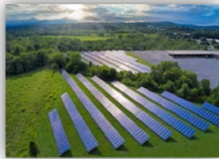
■ Asheville, NC System Size: 1.2 MWdc Commissioned in 2013
